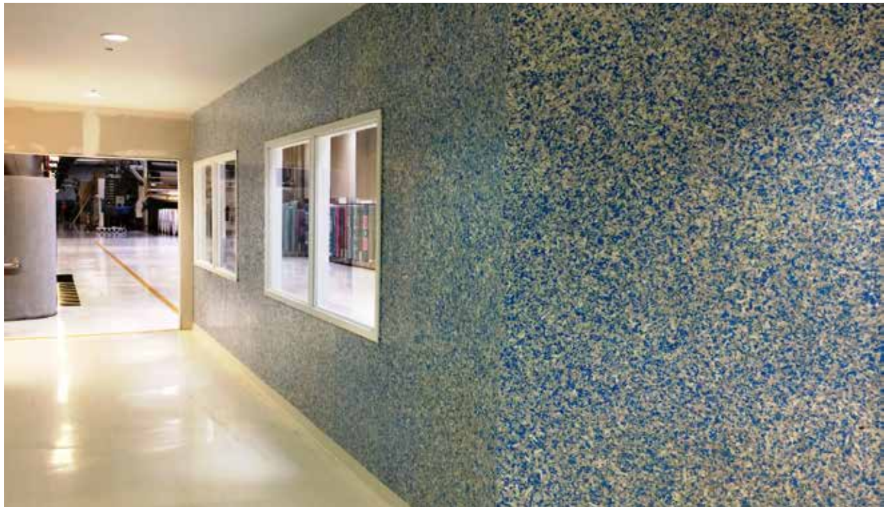
Manufactured by ReWall Company, the interior wall panels inside this plant are made from recycled paperboard beverage cartons via an innovative a specialized process that requires no water, formaldehyde glues or other hazardous chemicals.
